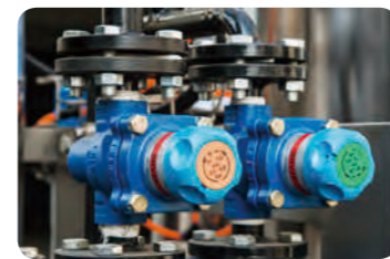
蒸汽减压阀 Steam Relief Valve
