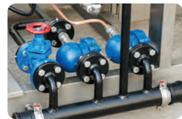
蒸汽疏水阀 Steam Drain Valve
